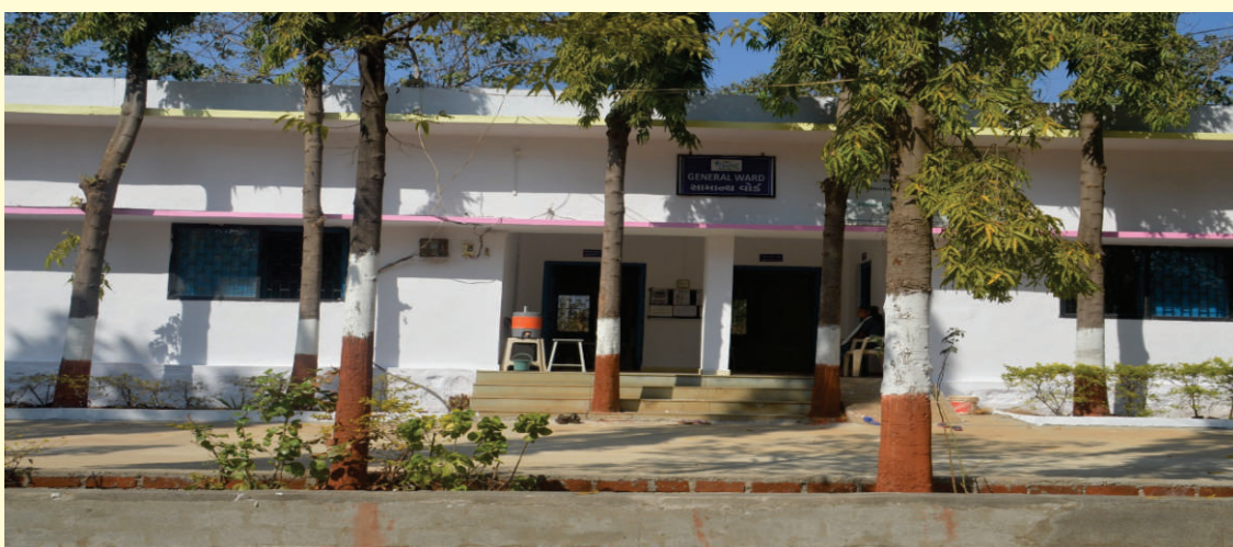
Front View of Narmada Hospital & Research Center (NHRC)
