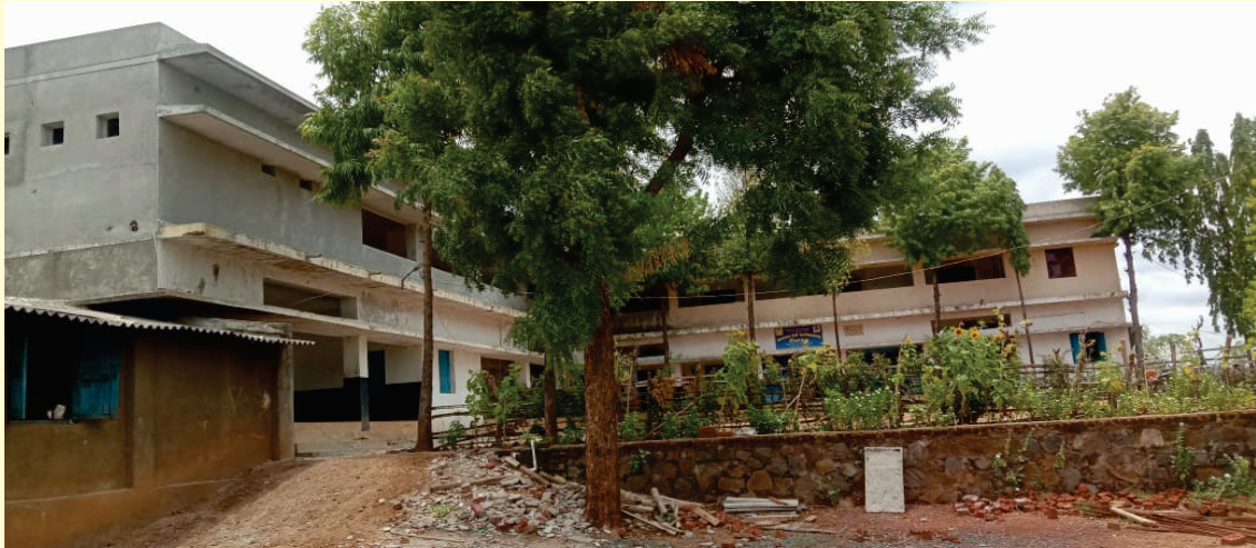
Lateral View Of Sanatan Dharm Ashram Shala
