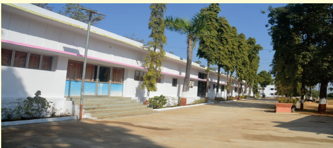
Internal View of Main Building of INRECA Sansthan
