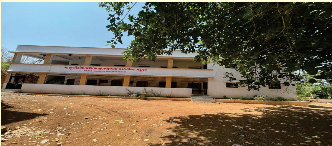
Vaidehi Kanya Ashram Shala New Building -2
